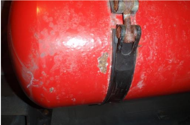
Fig.11.: At the inspection as “not usable” determined Type 1 cylinder under a CNG vehicle, because of the material corrosion. This type of failure can be detected well, if the vehicle inspection is regular and serious. In 2017 there was a wave to recall most of the VW CNG vehicles to check their bottles and had been replaced a large number of them. [Author]
